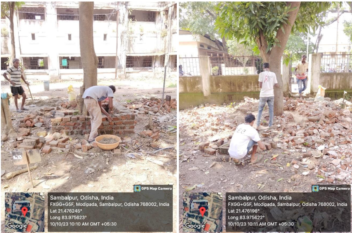
Construction & Demolition Wastes are using to develop sitting area under the tree
