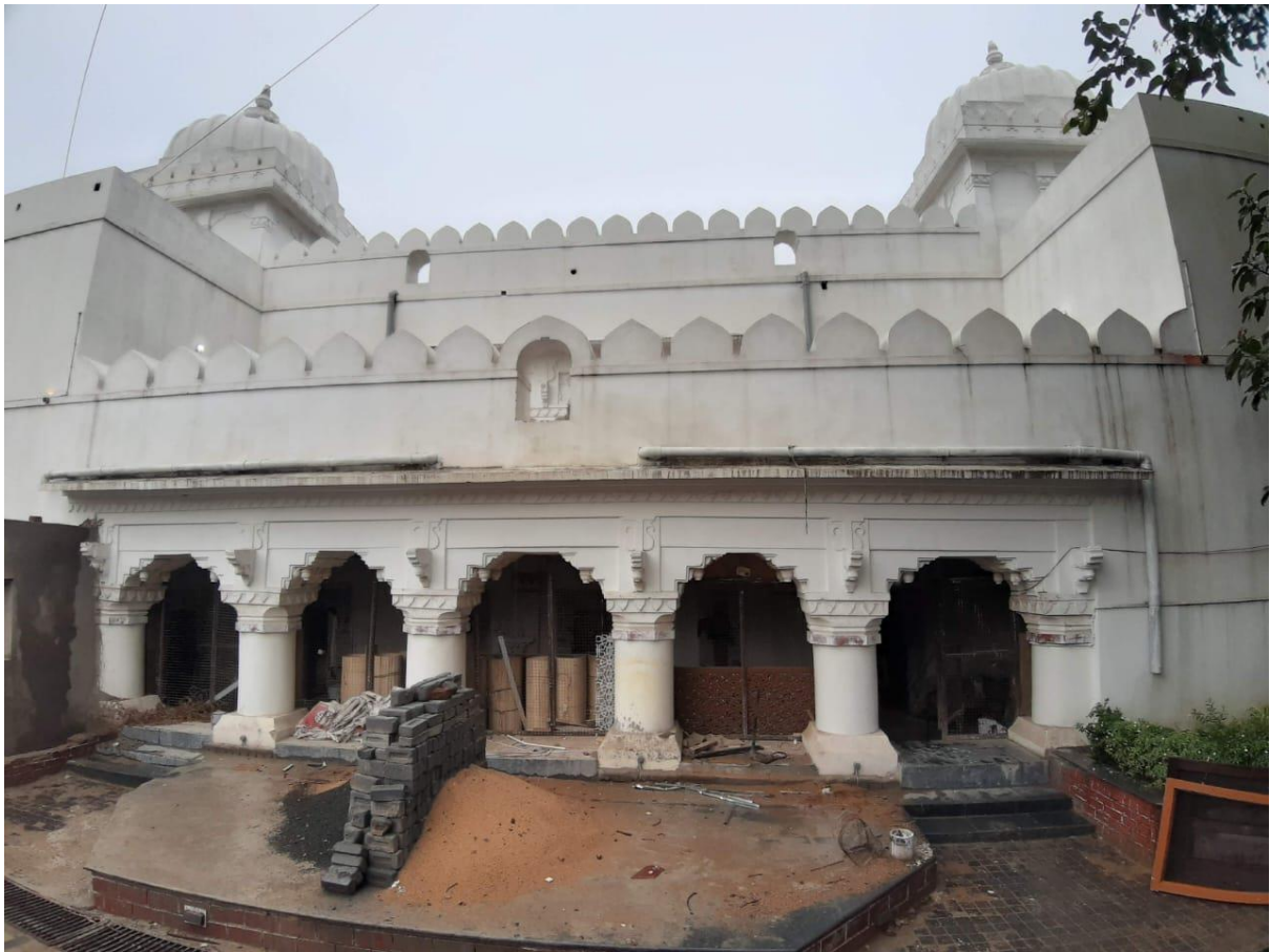
View of the Rani Bakhri(during the inspection )
