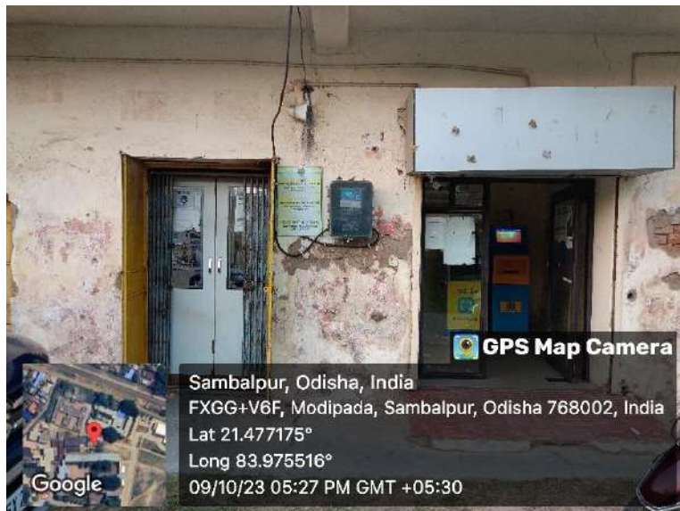
Banking & ATM facility at G.M. University, Sambalpur
